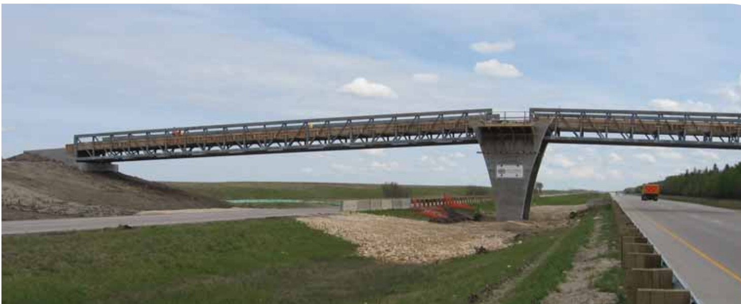
▲ A new pedestrian, bicycle and equestrian bridge across from the Birds Hill Provincial Park entrance lets people safely cross Highway 59.
